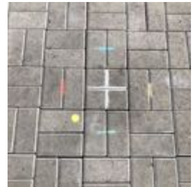
06. Roel Heremans art piece QTY: 1 63 x 63 x 5 cm Material: concrete blocks Location: Main hall
